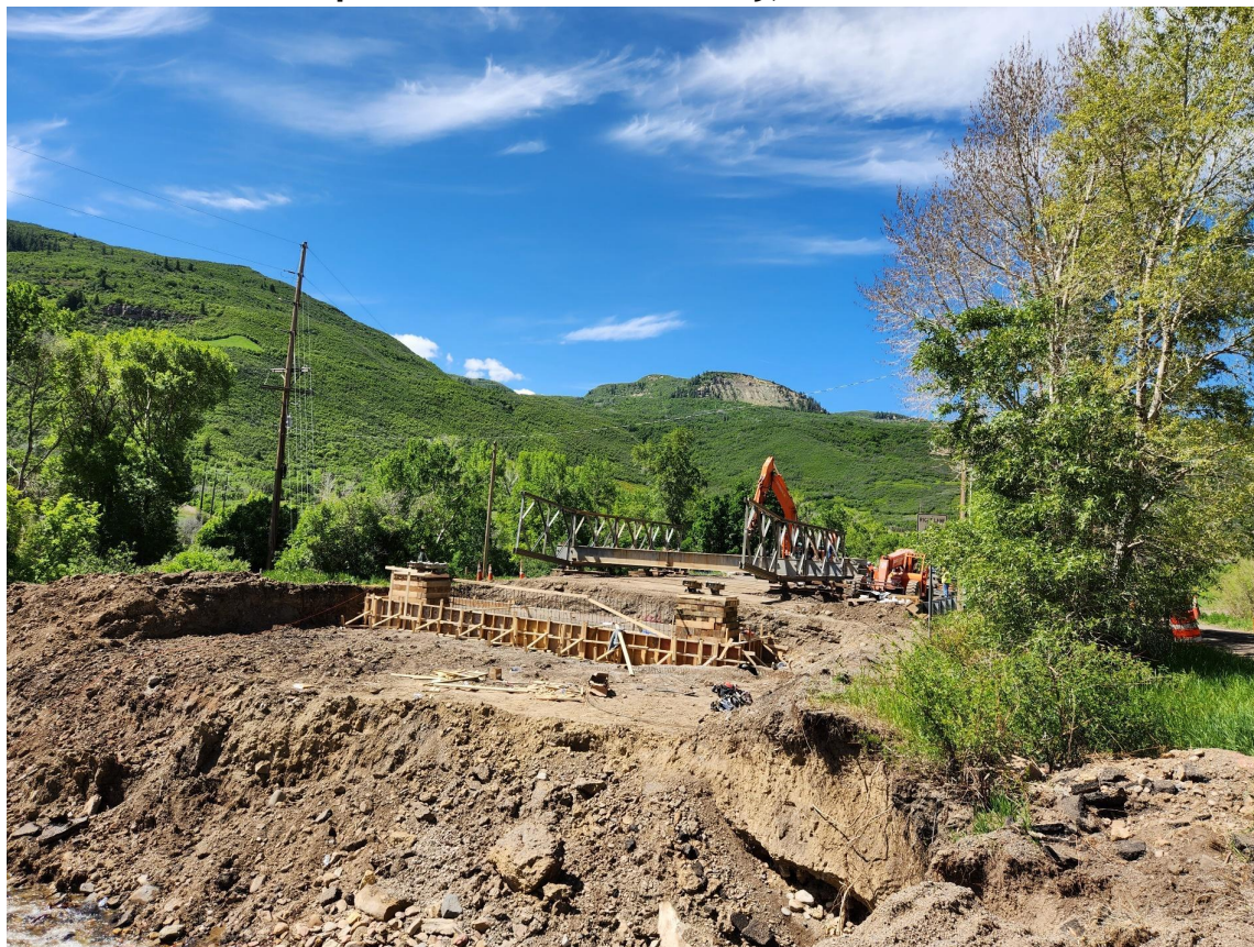
Temporary bridge starting to be assembled
