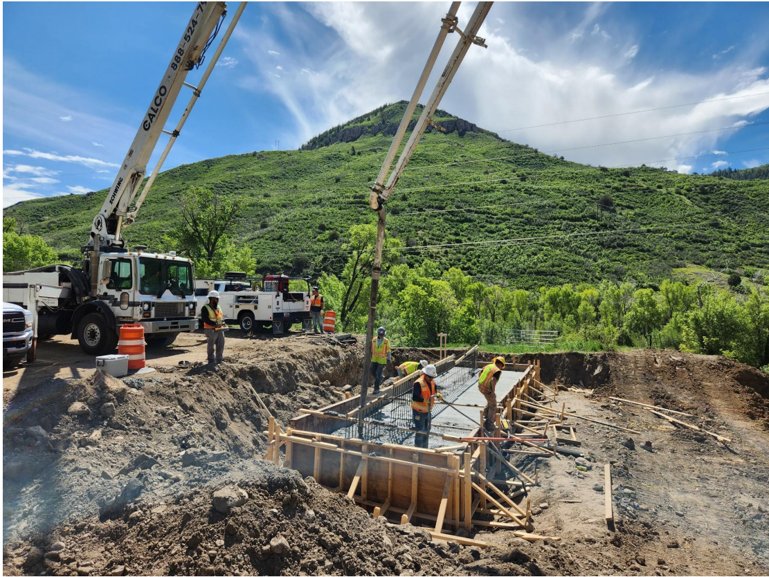
East side concrete pour for the temporary bridge foundation
